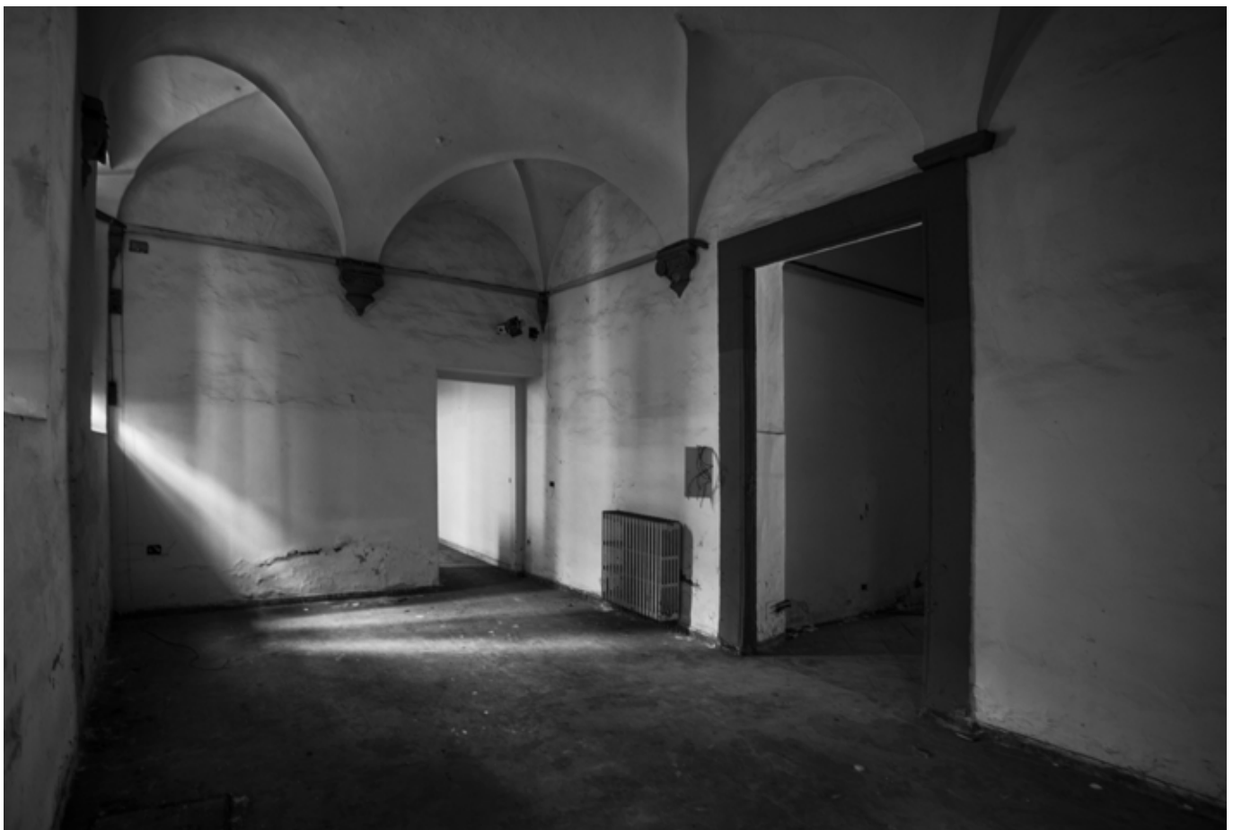
Vista interna / Inside view
