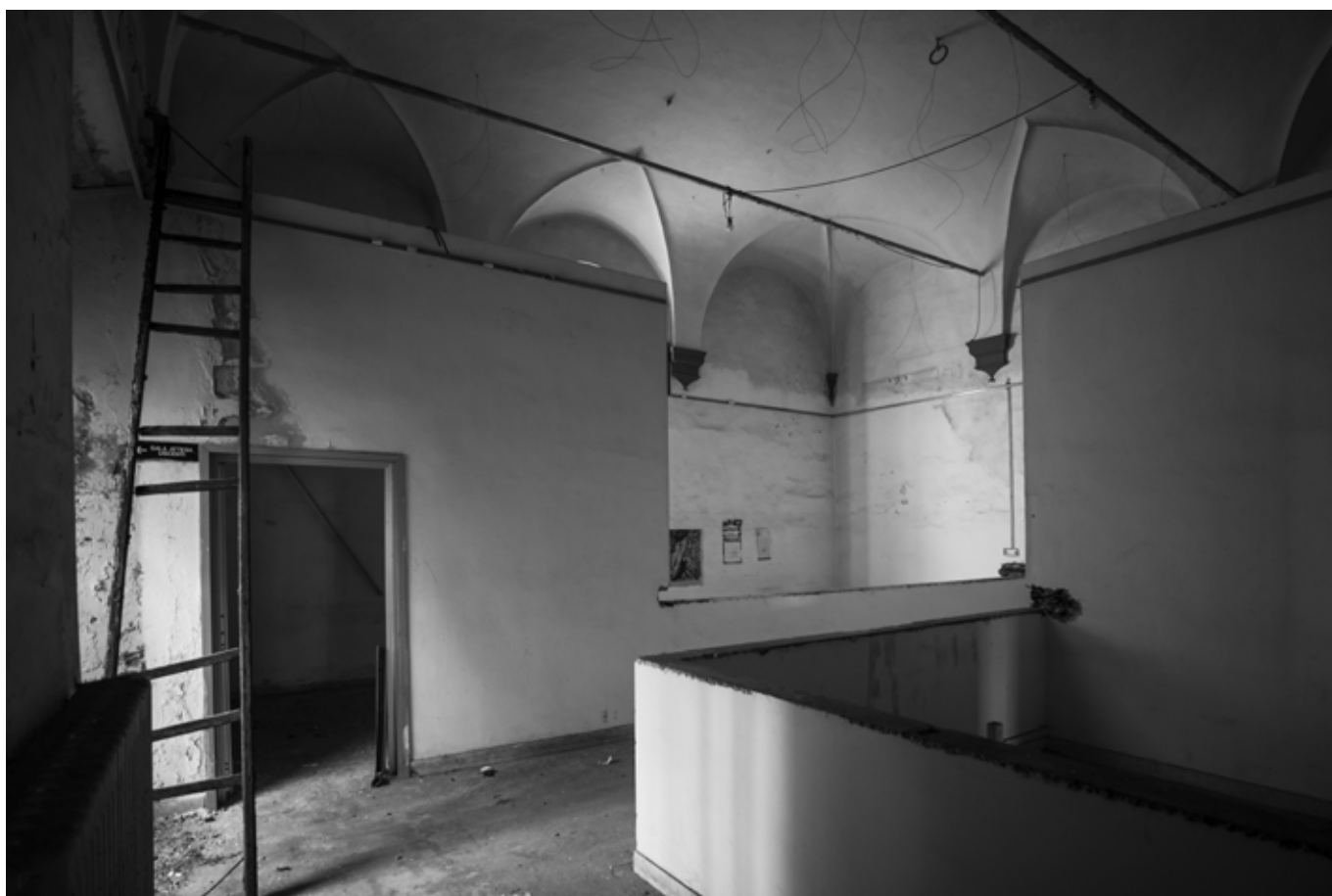
Vista interna / Inside view
