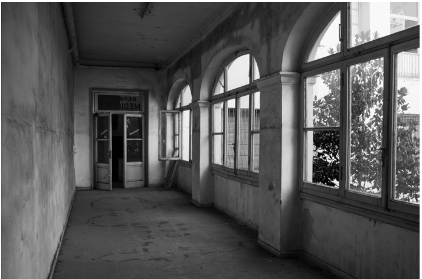
Vista interna / Inside view
