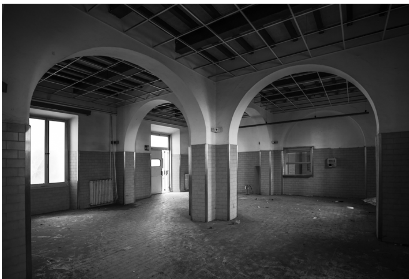
Vista interna / Inside view
