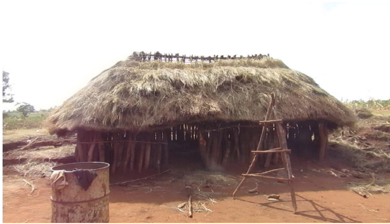
Hut: this one is being rebuilt. Dad is currently sleeping here.
